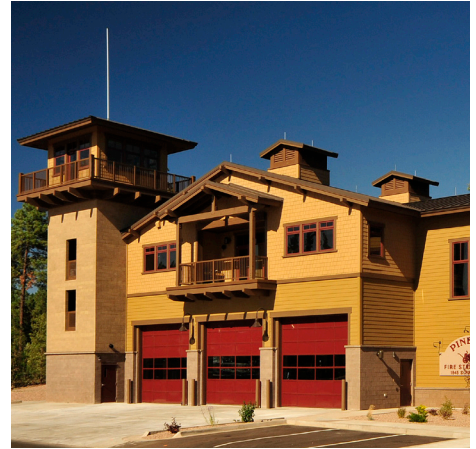
Pinetop Fire Station, Pinetop, AZ
