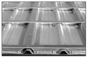
Note: If integral (fit under the HUGGERS) structural Sub-Rafters are provided, loosely place hats and HUGGERS in position prior to installing any fasteners to prevent alignment problems in these areas.
