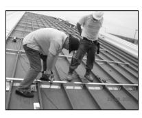
fasteners in addition to the clip fasteners or back lap the HUGGERS one full corrugation to produce a double thickness and continuity of the top flange across the lap.
