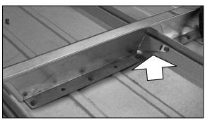
This arm prevents the ROOF HUGGER from rolling front to back under load and it is attached with a #17 fastener into the side of the existing panel high rib. Note that if the anti-roll tab is above the side of the existing high rib the ROOF HUGGER may not be pulled fully down into its correct position.
