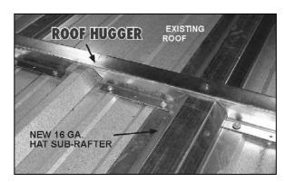
The Sub-Rafters will typically fit over the top of the major panel Ribs between 12"-24" centers. The Sub-Rafters will span from existing purlin to existing purlin and the ROOF HUGGERS will be placed on and into these members. The parts over the existing purlins will have 1/4"-14 T3 fasteners installed through the HUGGERS, through the Integral Sub-Rafter, through the existing roof panel and into the existing purlin. Oversize pre-drilling of the HUGGERS at Integral
