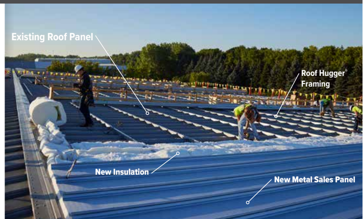
NEW METAL ROOF PANELS OVER EXISTING SLOPED METAL PANELS
