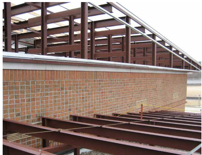
NEW METAL ROOF PANELS OVER EXISTING SLOPED METAL PANELS
